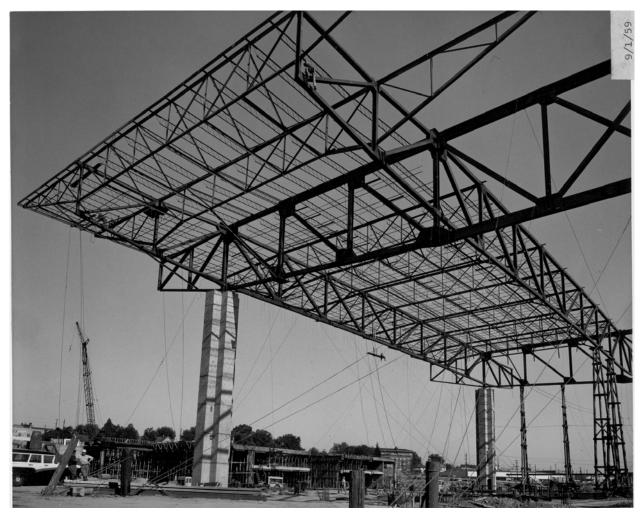
In fact, after the four columns were constructed, the steel truss roof was the first thing built for an elegantly simple reason. In the rain-soaked Northwest, the roof was built as an umbrella to
